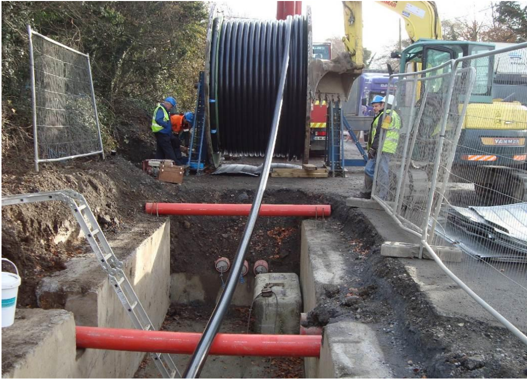
Figure 12 : HV cable pulling procedure (Standard drum set-up)
