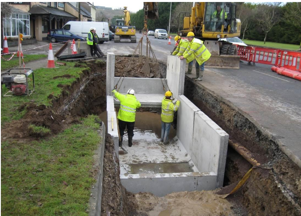
Figure 11 :Standard joint bay under construction (pre-cast)
