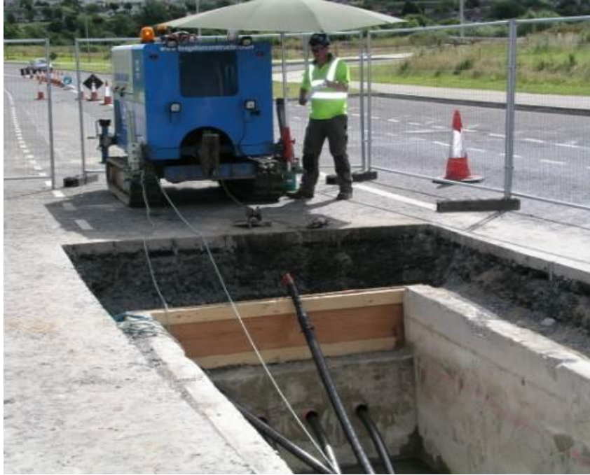
Figure 14 : HV cable pulling procedure (Standard pulling winch set-up)
