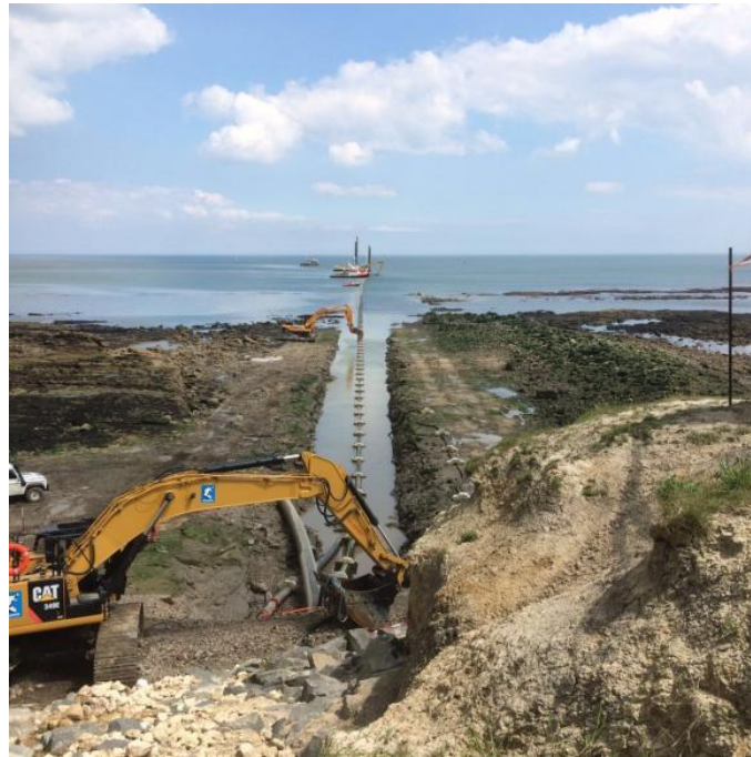
Figure 17 Photo Installation of Cable Trench at Landfall Location
