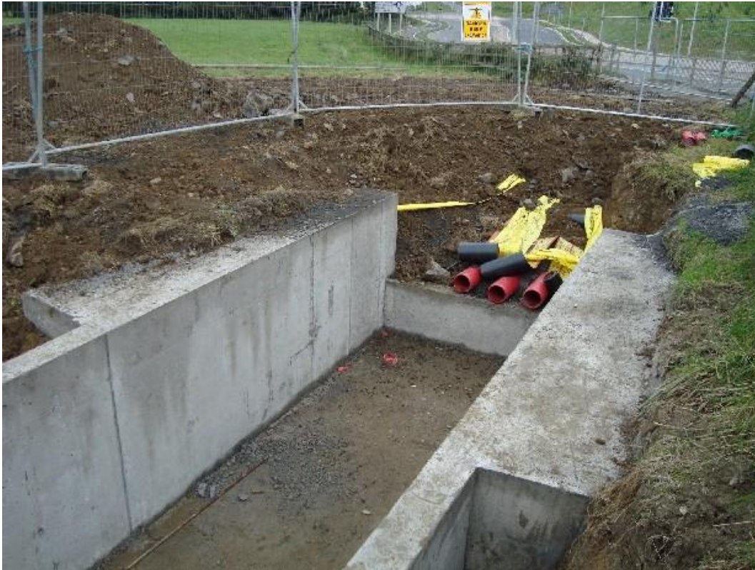
Figure 10 : Completed joint bay prior to cable installation (in-situ)
