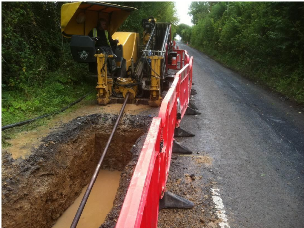
Figure 6: HDD rig set up on regional road.
