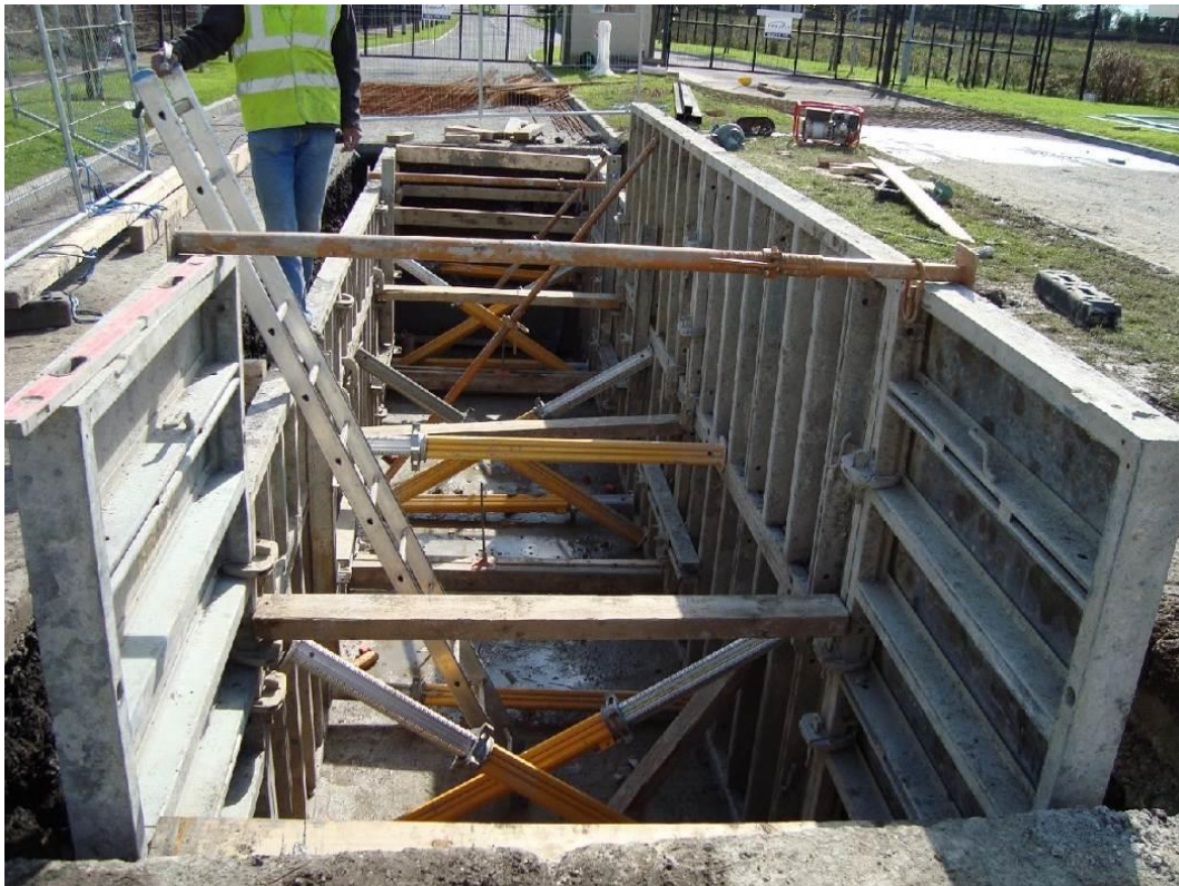
Figure 9 : Standard Joint Bay Under Construction (in-situ)
