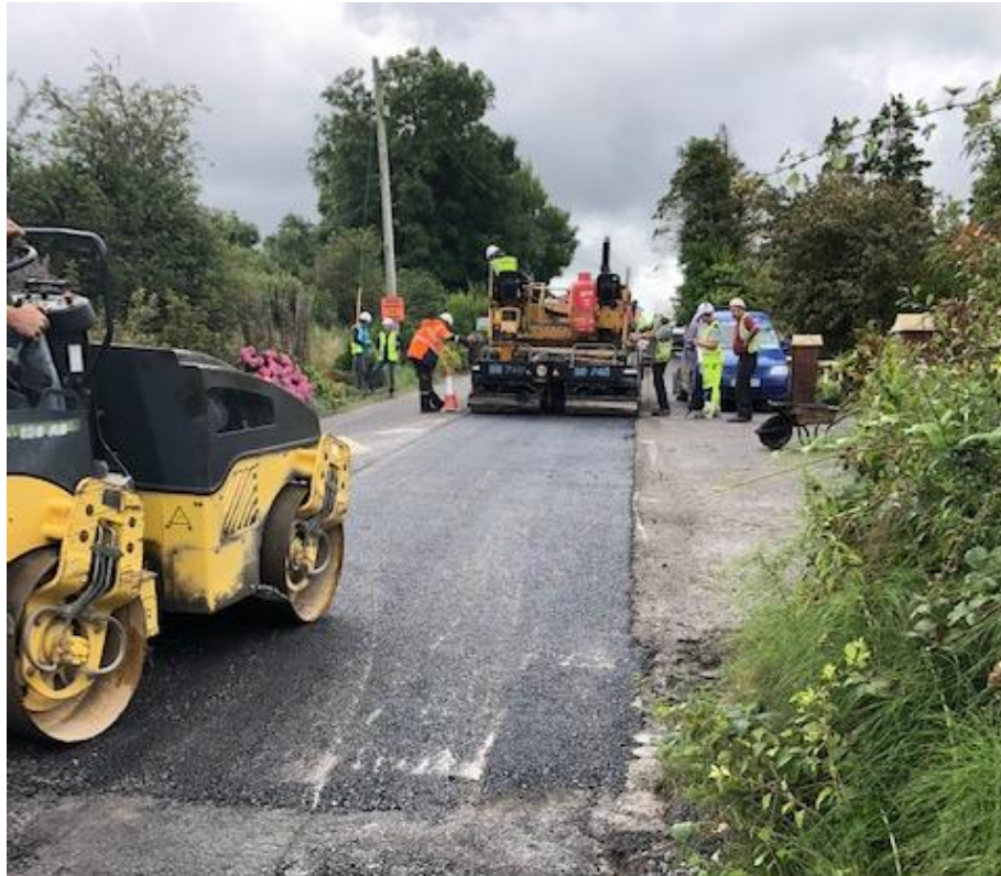
Figure 2 : Permanent Reinstatement of road surface over trench
